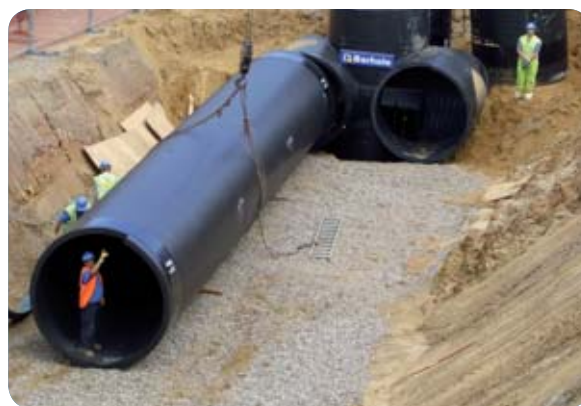
↑ A huge sewer pipe being laid in Cromer
